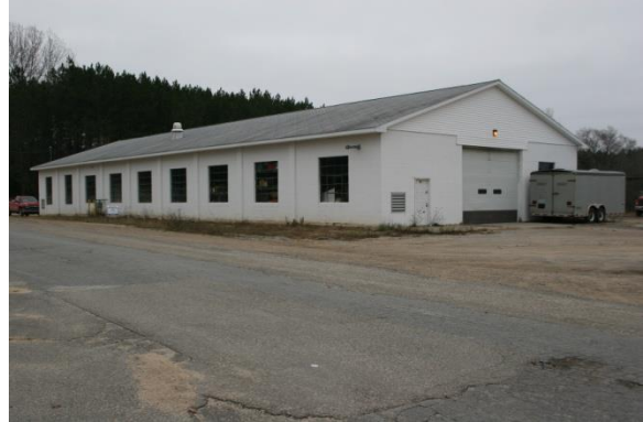
Osceola County Road Commission Garage Tustin, Michigan
