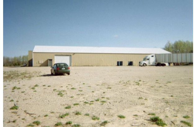
Krauter Forest Products Facility Ashton (Lincoln Township), Michigan
