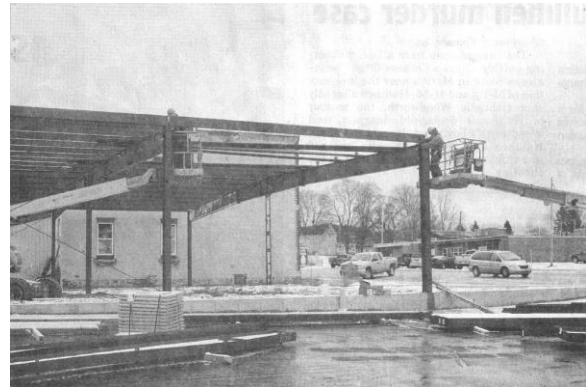
Dollar General Store Under Construction Tustin, Michigan
